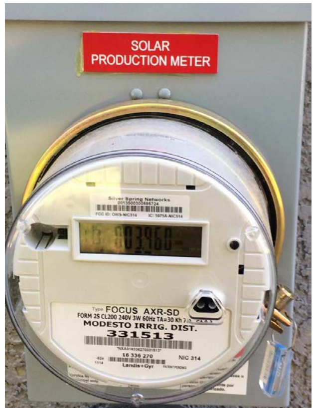
Figure 4: Solar Production Placard
