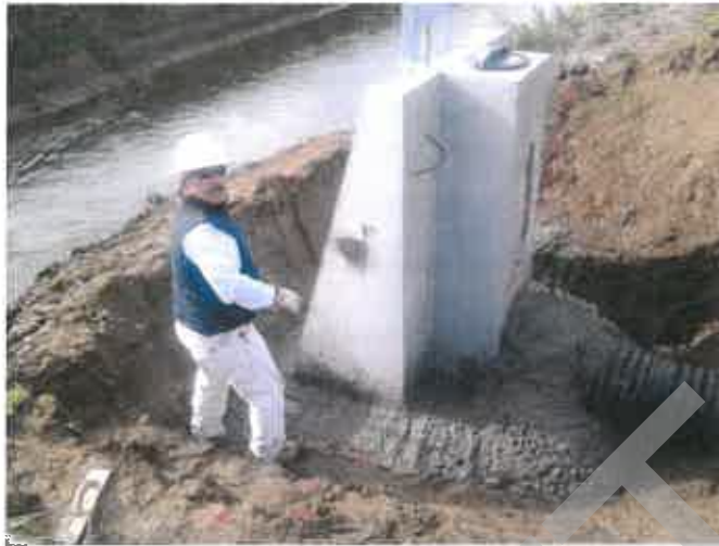
Figure B-15. Installation of GCID meter gate
