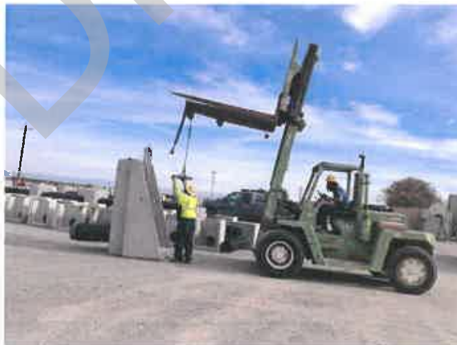
Figure B-14. Pre-cast metergate ready for transport
