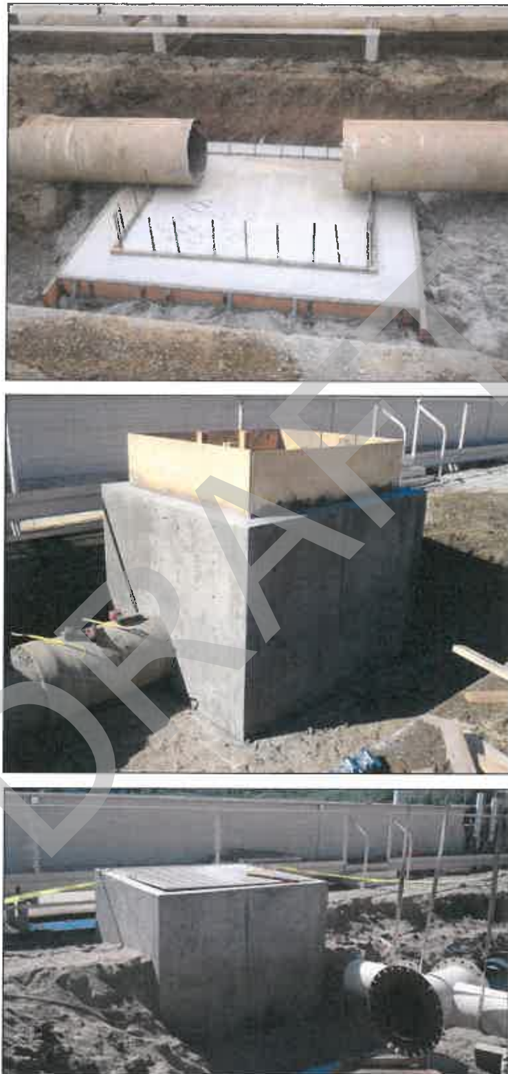
Figure A-2. Construction of the drain pipe connection box (right). Students in BRAE 433 (Fall Quarter) helped design and construct the bottom concrete slab shown in the top photo.
