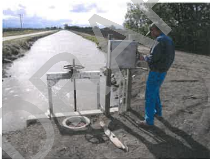
Figure B-12. Large diameter stilling well, with cover to minimize having it fill with dirt from the road. Strong concrete, with the rim of the stilling well at the same elevation as the bulkhead top.
