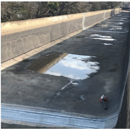
SEALED ALL SIX JOINTS AT THE DRY CREEK FLUME
