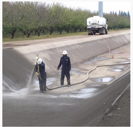
SPRAYED 3,500 CUBIC-YARDS OF GUNITE FOR CANAL LINING
